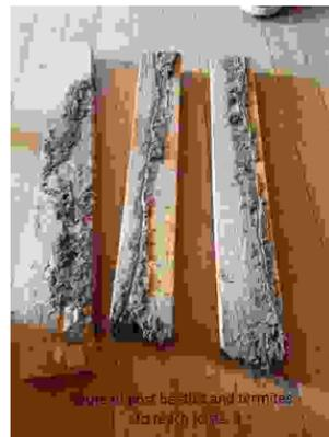
Signs of post beetles and termites damage to joists
