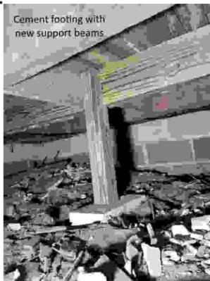
Cement footing with new support beams
